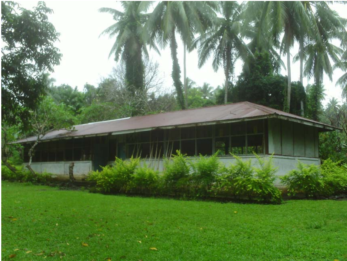
Figure iii. Another earlier classrooms (Current Grade 6 classrooms)
