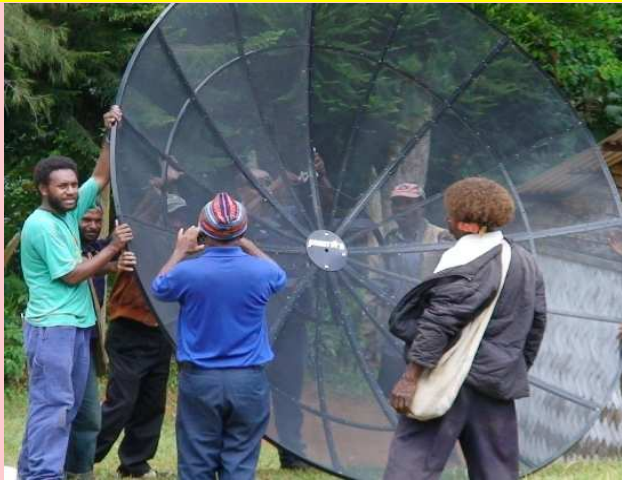
Staff of the National Education Media Centre install a satellite dish at Walete Primary School with the help of locals.
